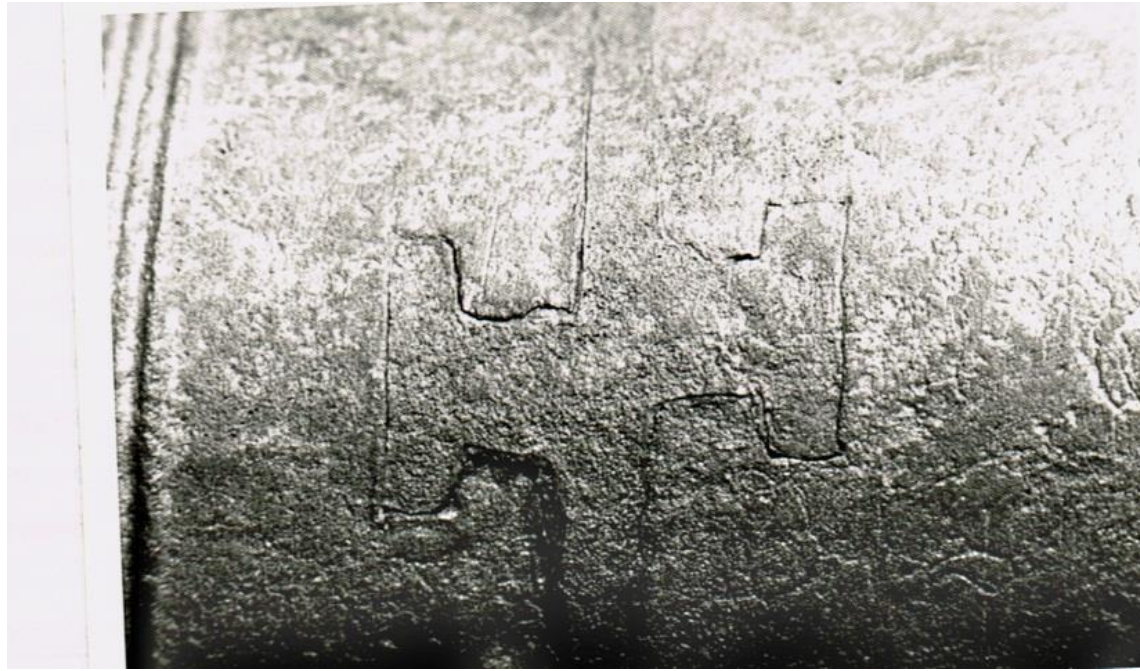
Plate 4.4(b): A typical Meander Joint
